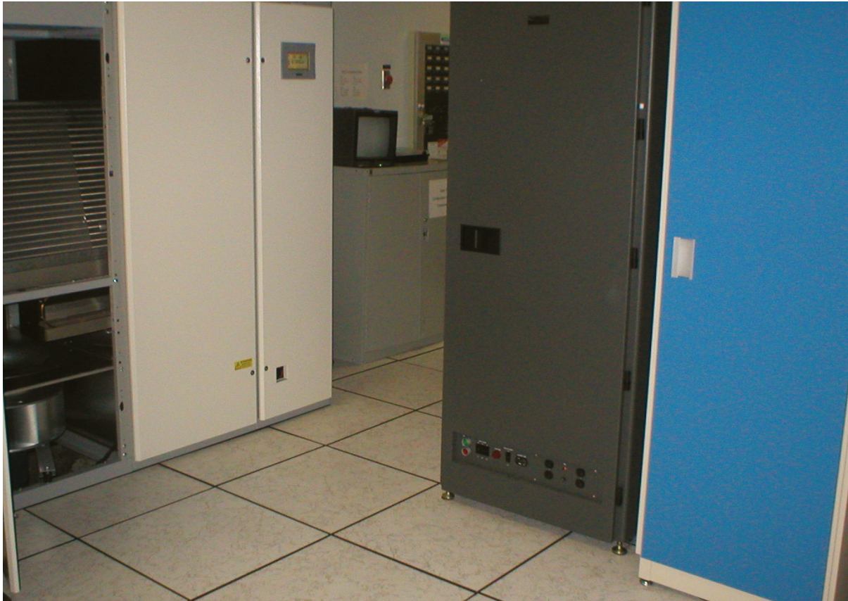
The “hot spot” began with the server only 3 feet away and extended to an area 12 feet away.
